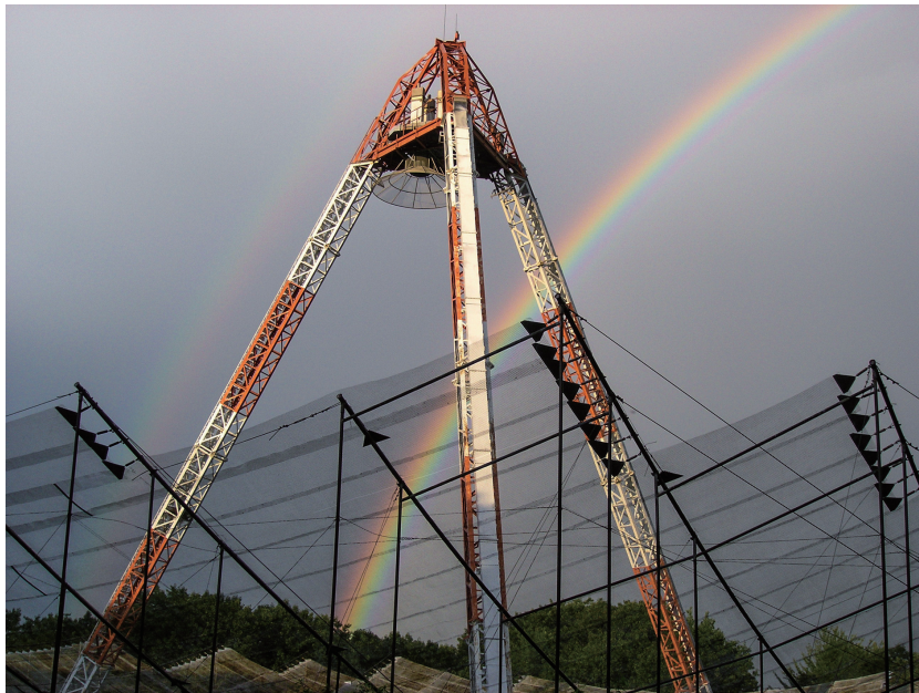
Figure 4. The incoherent scatter radar (ISR) at Millstone Hill, located near Boston, Massachusetts, and operated by MIT Haystack Observatory, is a Class-I large geospace facility funded by the US National Science Foundation. Shown is the larger 68-meter diameter zenith antenna used by Millstone Hill for vertical ionospheric measurements. Using this antenna in combination with a fully steerable 46-meter diameter antenna (not shown), the radar measures multiple ionospheric plasma state parameters over a broad section of the eastern US and a wide altitude range. These parameters include electron density, ion and electron temperatures, and plasma velocity. Millstone Hill ISR conducted experiments during the 2017 eclipse to probe ionospheric changes. Photo by Shun-Rong Zhang.
